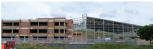
RIVERHORSE VALLEY WAREHOUSE, OFFICE BLOCK & SUBSTATION
